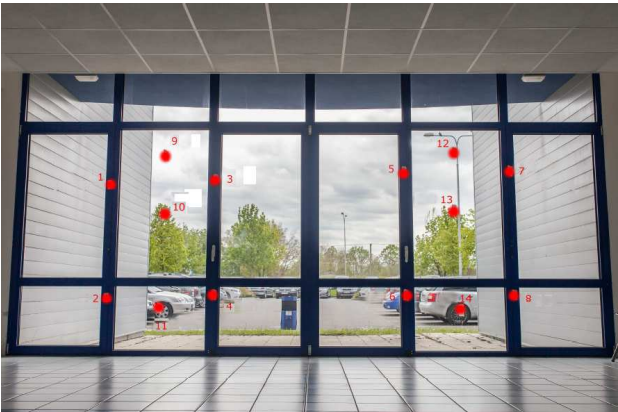
Fig. 2. Configuration of measuring points in the 1st floor corridor (S).
