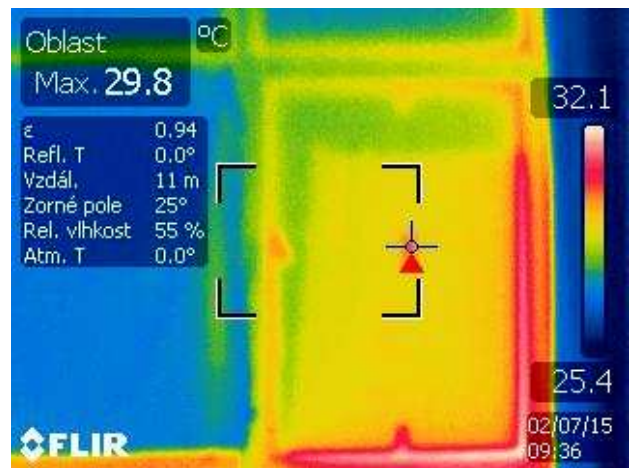
Fig. 4. Sample thermogram (3 rd floor, room EL311 - S).
