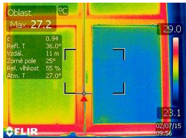
Fig. 5. Sample thermogram (5 th floor, room EL511 - S).
