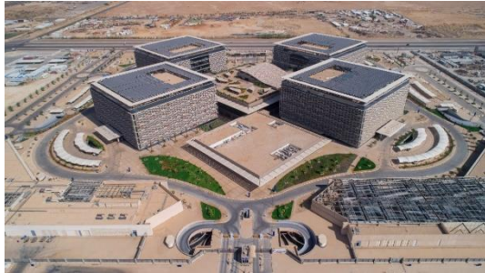
Fig. 1 View of installed rooftop PV
