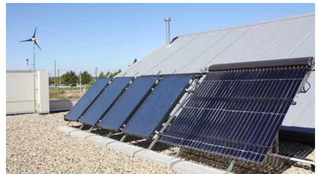
Fig. 6. External set of RES devices: PVT, ETC, microwind turbine.
