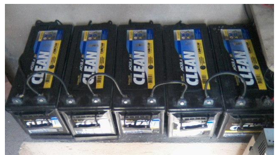
Figure 06: Battery Bank
