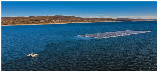
Fig. 2 . FSPV System in Dam Rabagão
