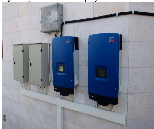
Fig.2. Out-door Sunny Tripower Inverter
