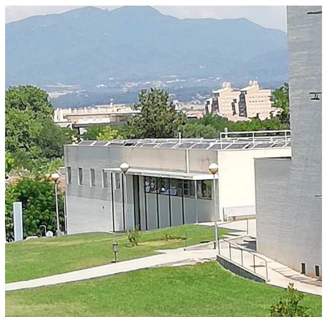
Fig. 4. PV cells placed at the roof of P1 labs
