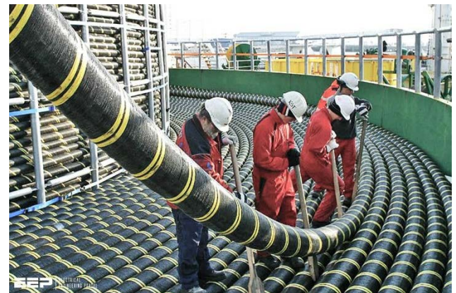
Fig. 2. HVDC submarine power cables.
