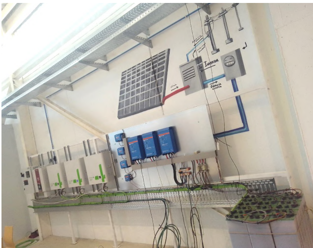
Fig. 8. Connection of the wind turbines to the battery bank.
