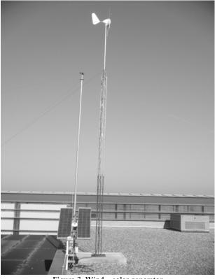
Figure 3. Wind - solar generator
