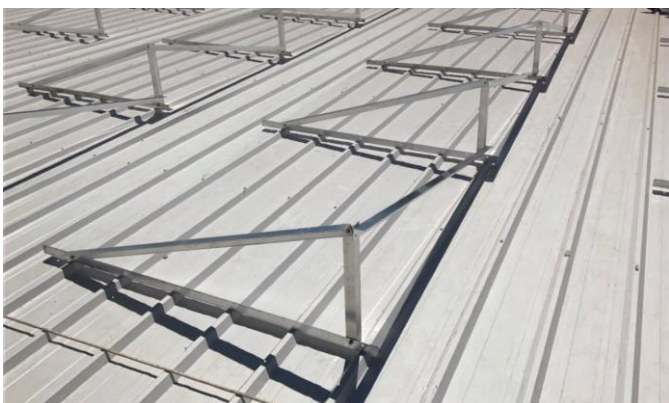
Fig. 4 Aluminum supports for photovoltaic panels.
