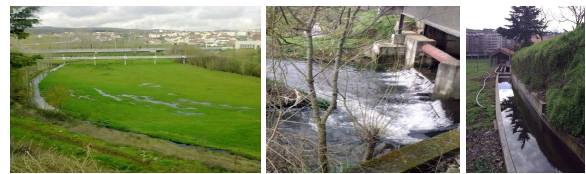
Fig. 1. Irrigation canal in the IPB Campus (left), small intake weir in Fervença river (centre) and the end of feeder canal (right).
