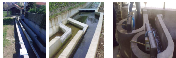
Fig. 3. Feeder canals (left), discharge divisor and spillway (centre) and turbine supporting structures (right).
