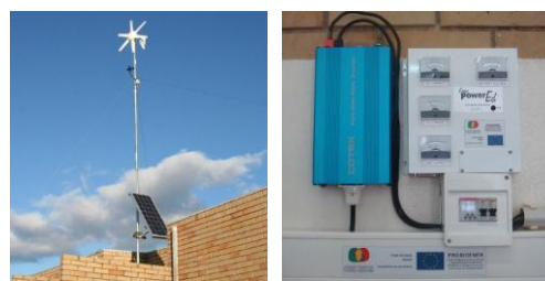
Fig. 8. Hybrid system combining solar PV and wind energy.
