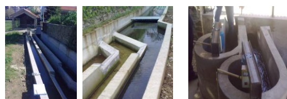
Fig. 5. Water canals (at left), zone of overflow (in center) and turbines in the "snails" (at right).
