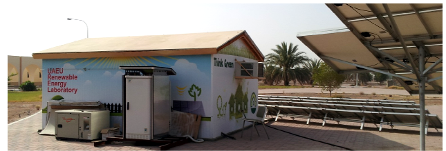
Figure 3 UAE University Renewable Energy Laboratory
