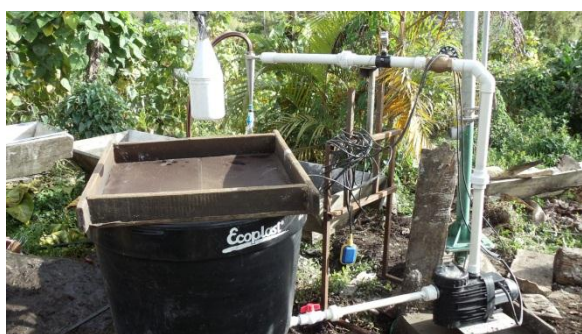
Fig.12. Installation of the solar pump and the hydrocyclonic system in Pasca (Cundinamarca).
