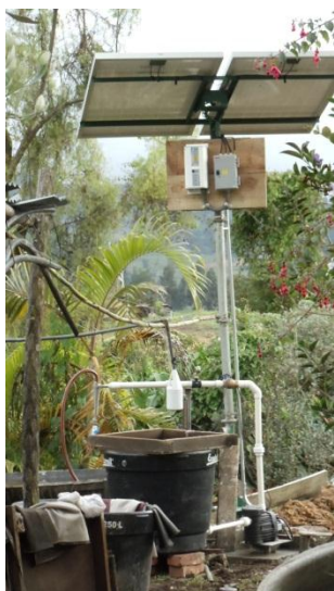
Fig.13. Panoramic view of the hydrocyclonic system (down) and photovoltaic system (up) connected together.
