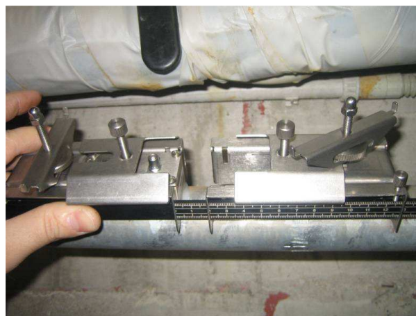
Fig. 2. Installation of flow meter
