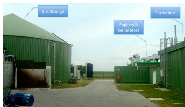
Fig.1: Layout of the biogas power plant's main components.
