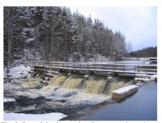
Fig. 2. Part of the dam at the pilot power plant, picture taken 29<sup>th</sup> November 2007. The generator pool is on the right (partially visible). As can be seen, the hydrological situation is such that the inflow is greater than the plant's capacity, and the spillage is high.
