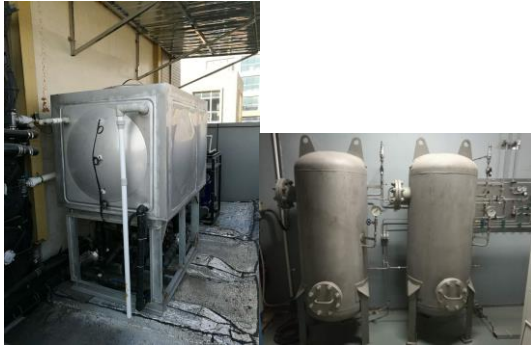
Fig. 7. Hot water tank (L) and Main hydrogen storage tanks (R)
