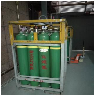
Fig. 8. Spare hydrogen storage tanks
