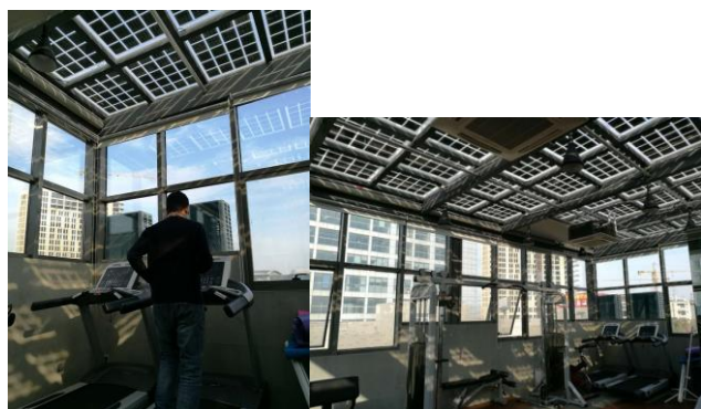
Fig. 5. GYM with photovoltaic panel roof
