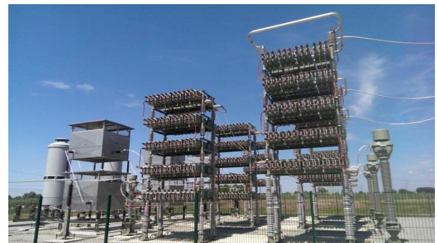
Fig. 1: Photo of a Mechanically Switched Capacitor with Damping Network connected to the German 380-kV-network.
