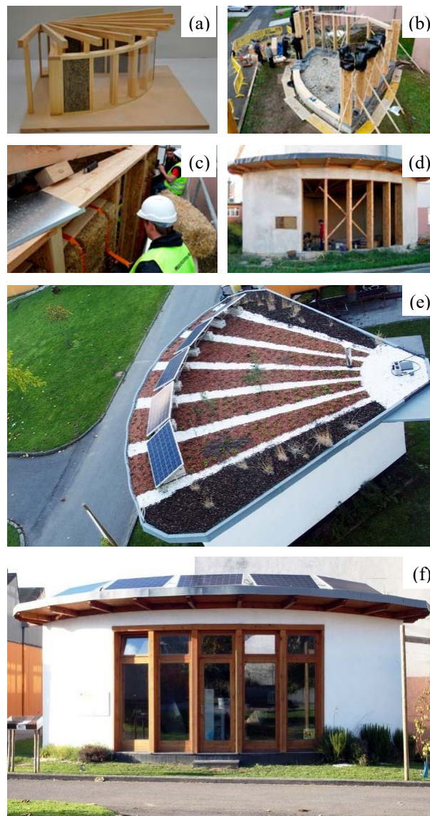
Figure 2. Bioclimatic module “A Vieira” design and construction process: a) Model design, b) Foundations, c) Walls construction, d) Module without enclosures, e) Green roof, f) Module finished look
