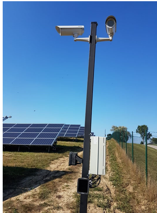
Fig.6: Uniview camera and lamp mounted over a pole for CCTV surveillance, I+D Energías, Poland
