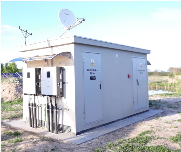
Fig.4: Satellite Antenna mounted on the top of the transformer station
