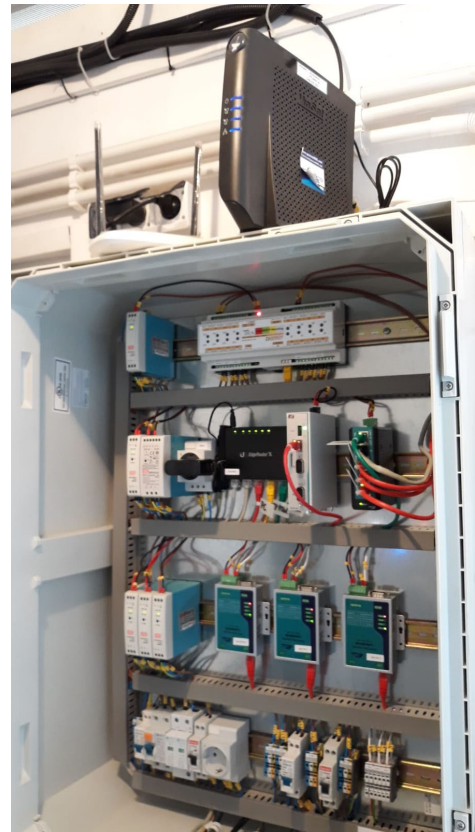
Fig. 3: Satellite Modem and Router already connected to the monitoring cabinet, inside transformer station.
