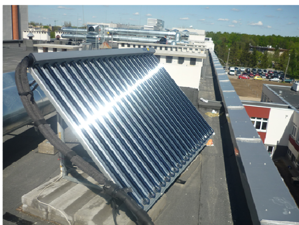
Fig.1. Solar collector on the roof (source: D. Krawczyk)
