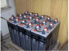
Figure 9-Batteries used as load
