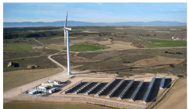
Fig.2. Hybrid power plant with a wind generator, solar photovoltaic panels and backup diesel generators [2].
